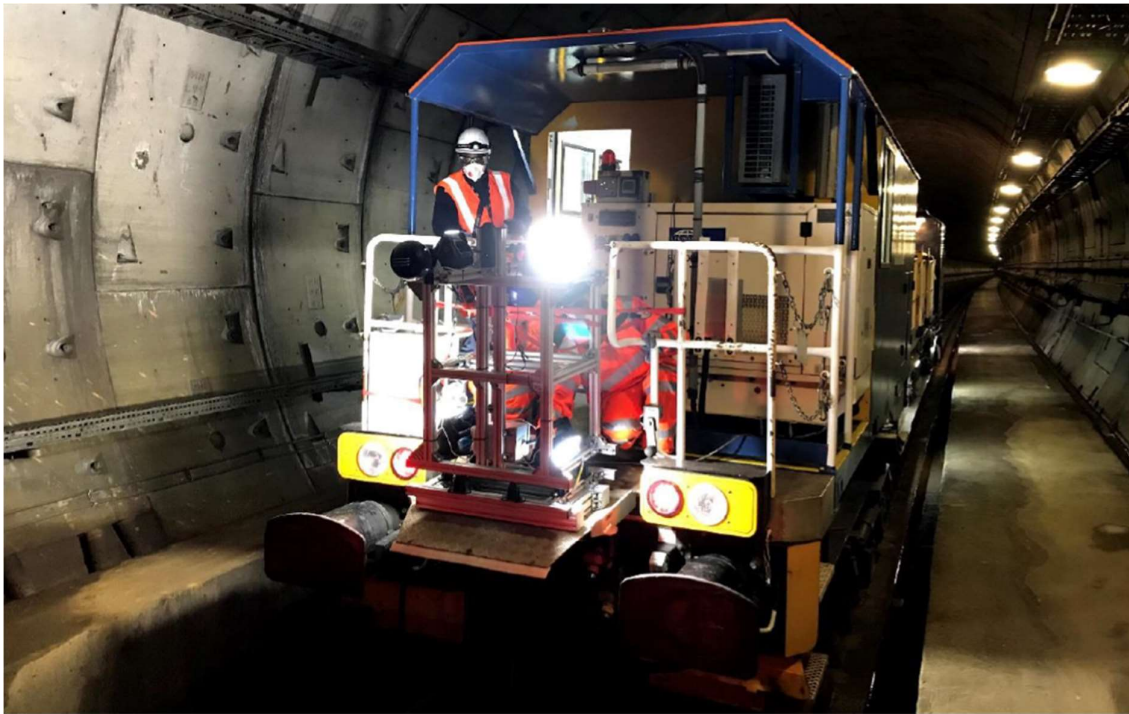
Figure 15 – The MPV with the Tunnel Vision equipment installed recording tunnel condition
