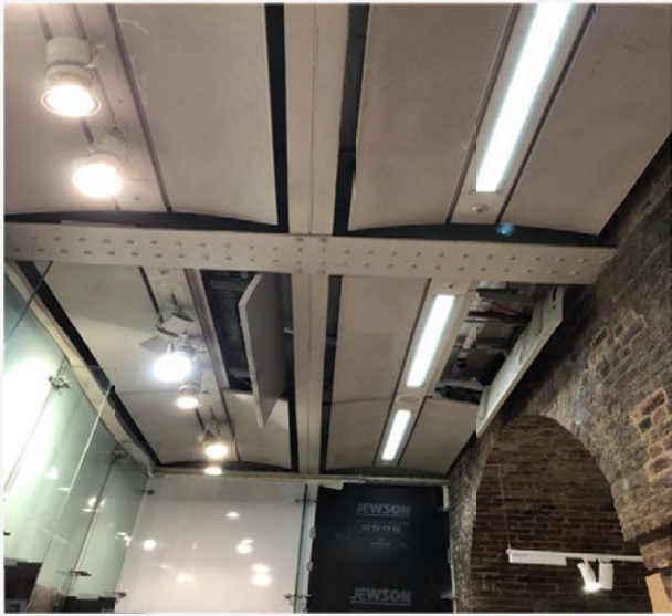
04 IMAGE OF EXISTING METAL CEILING
